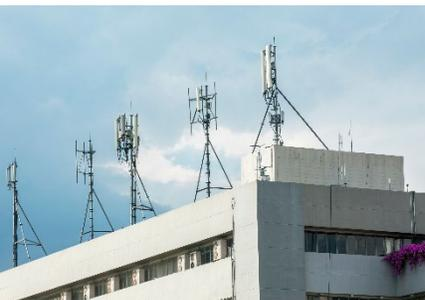
5G small cells can be millimeter wave (mmWave) or Sub-6GHz. mmWave uses high-frequency bands that offers faster speeds but at a much shorter range and with limited propagation—high-frequency signals are easily blocked by doors, windows, trees, and walls. In contrast, Sub-6 uses mid-to-low frequencies bands at reduced speeds but with far better
